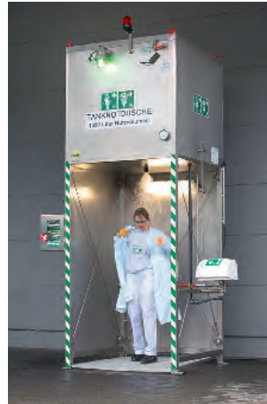
Tanknotduschen Tank safety showers
