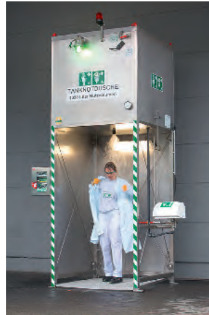
Tanknotduschen Tank safety showers
